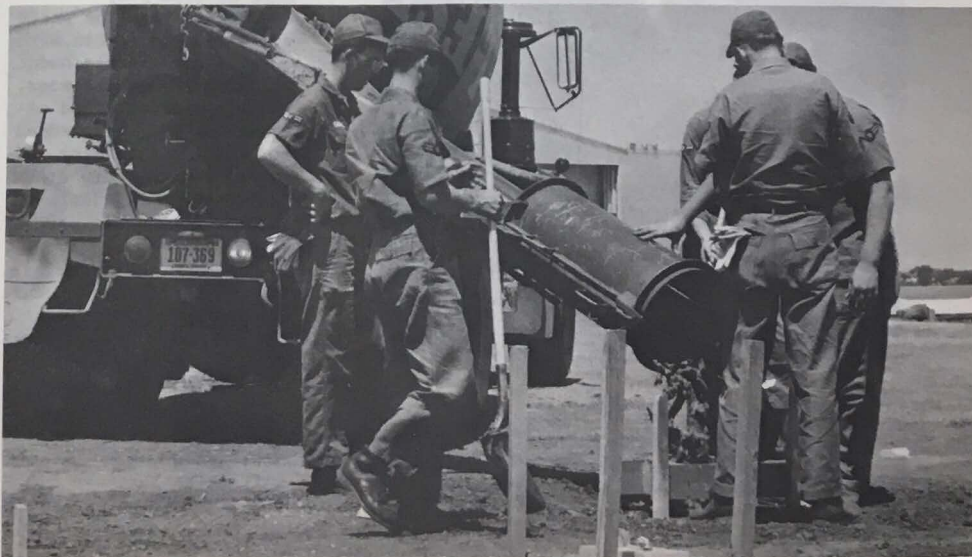
Civil engineers of the 937th pours concrete for two butler buildings.
